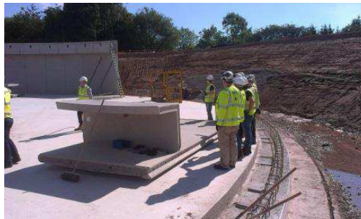
Wall Unit (with integral launder channel) – Prior to Installation
