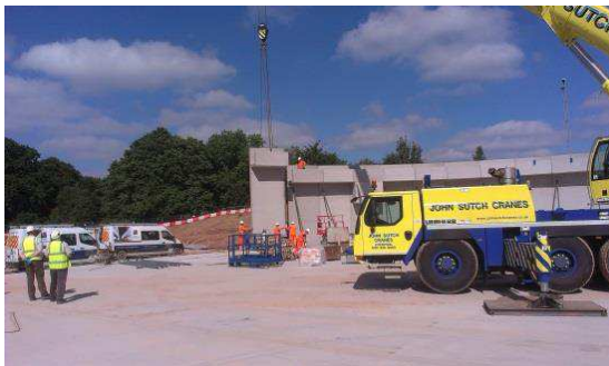
Wall Unit – Lifting into position and Placement
