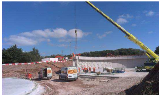
Wall Unit – Lifting into position and Placement
